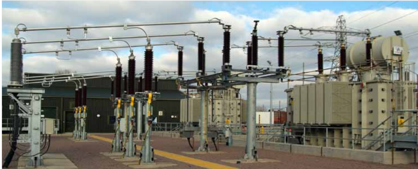
The completed Sheringham Shore onshore station at Salle.
